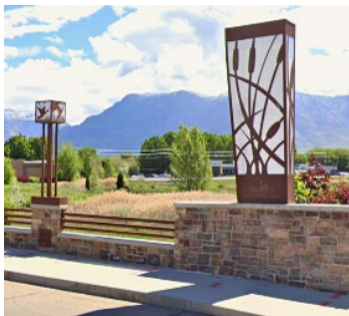
Image 14: Bridge in American Fork, UT
