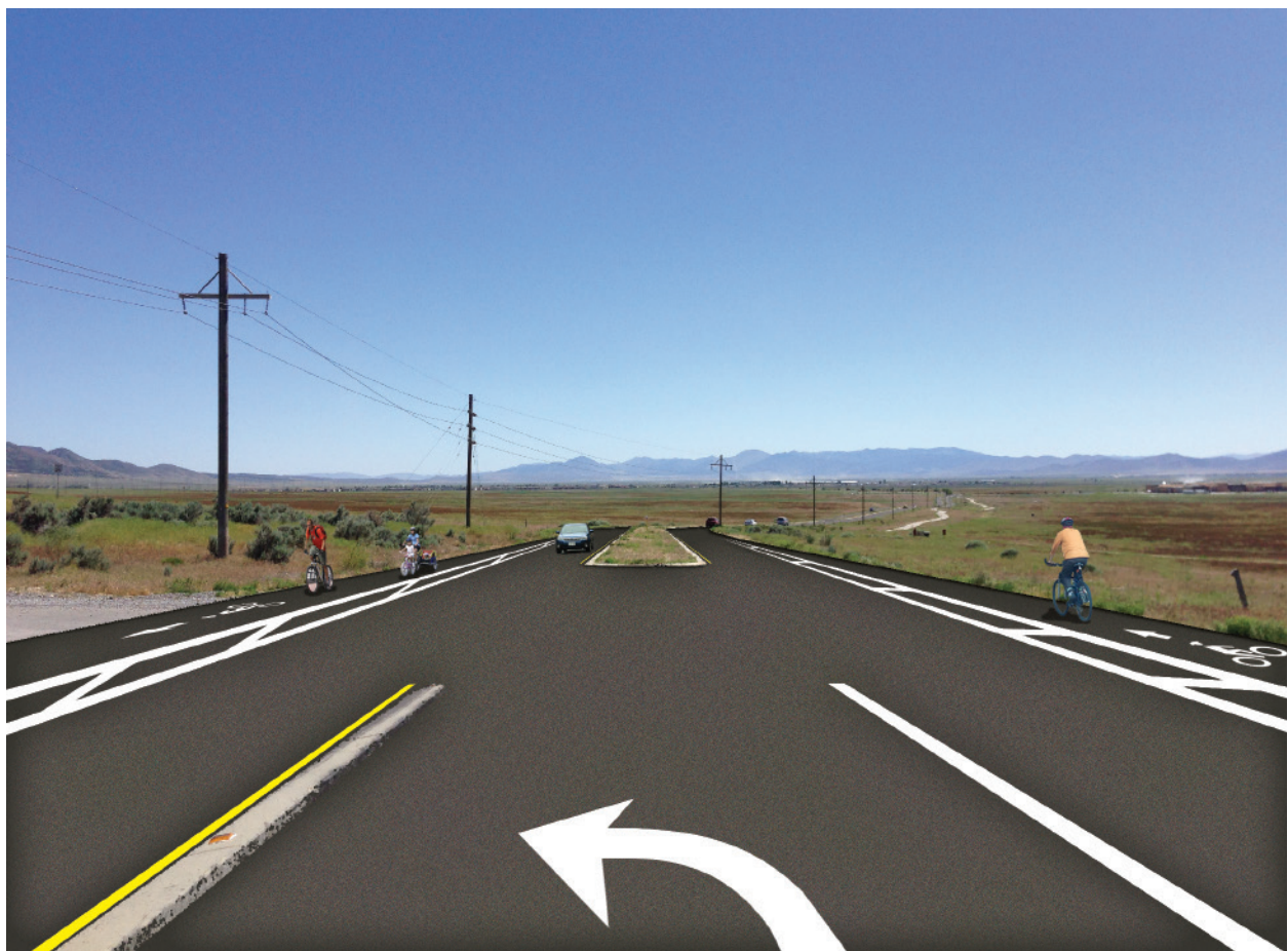
A rendering of what Pony Express Parkway would look like south of Unity Pass, with improved shoulders and buffered bike lanes
