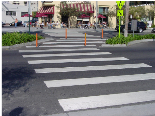
Median refuge island
