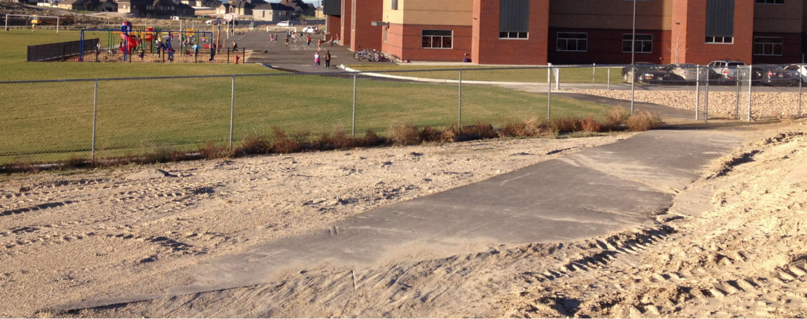
Dirt from adjacent development on a shared-use path leading to Black Ridge Elementary
