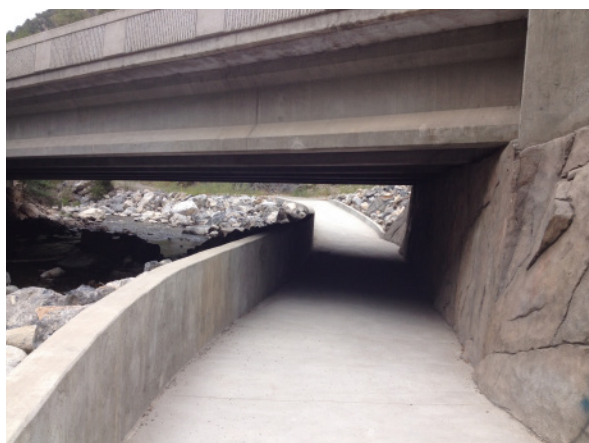
A grade-separated undercrossing using the existing slope and riverbed to pass under a roadway
