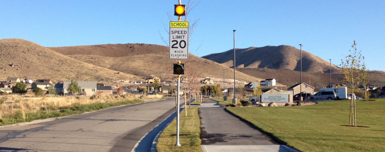
School zone speed limit sign and yellow flashing beacons in front of Black Ridge Elementary School
