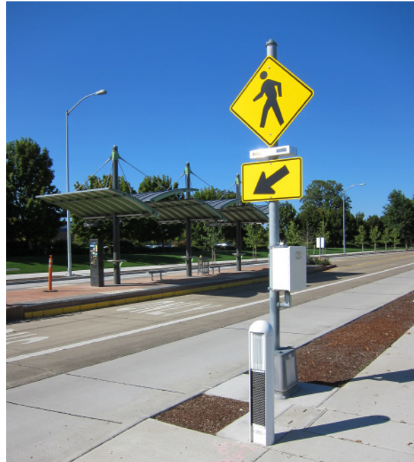
RRFB with passive detection (white bollard in foreground)
