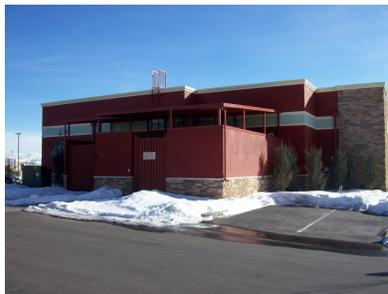
**Screening for mechanical equipment matches building in material and color**
