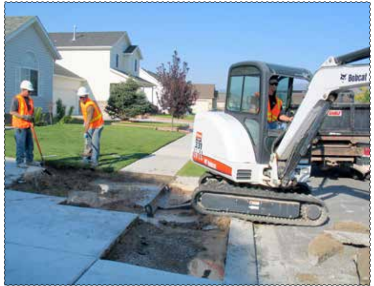
The Water Department repairs a ruptured pipe
