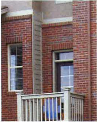
Examples of poor masonry design: "Floating" masonry (top photo); Brick termination at outside corner (bottom photo)
