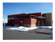
Screening for mechanical equipment matches building in material and color
