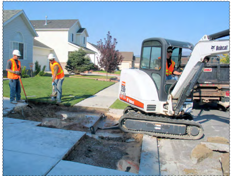
The Water Department repairs a ruptured pipe
