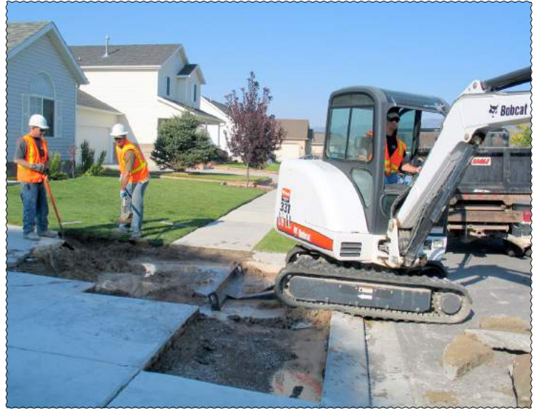
The Water Department repairs a ruptured pipe
