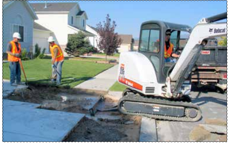
The Water Department repairs a ruptured pipe
